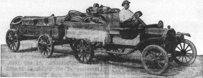
Pulling a 5-Ton Load—3 Tons on Ford and Two Tons on Trailer.
