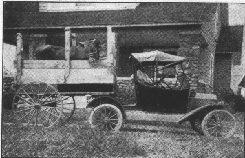
Roadster and Trailer Coupled Together by a Fifth Wheel Attachment.
