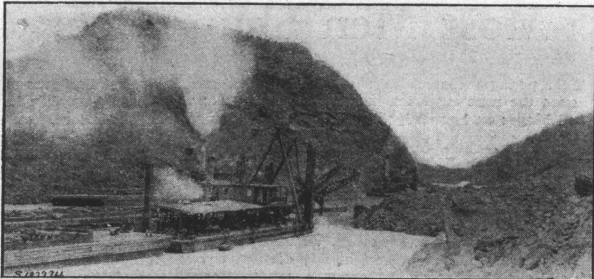
Panama Canal Almost Completely Blocked by Successive Land Slides North of Gold Hill.
