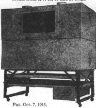
Greatest improvement in Smoke Houses. Smoke cooled by air and radiation. Works automatically. The faster the fire burns, the faster the cool air is drawn through ventilation holes to cool the smoke. Get any heat you desire by adjusting ventilators
