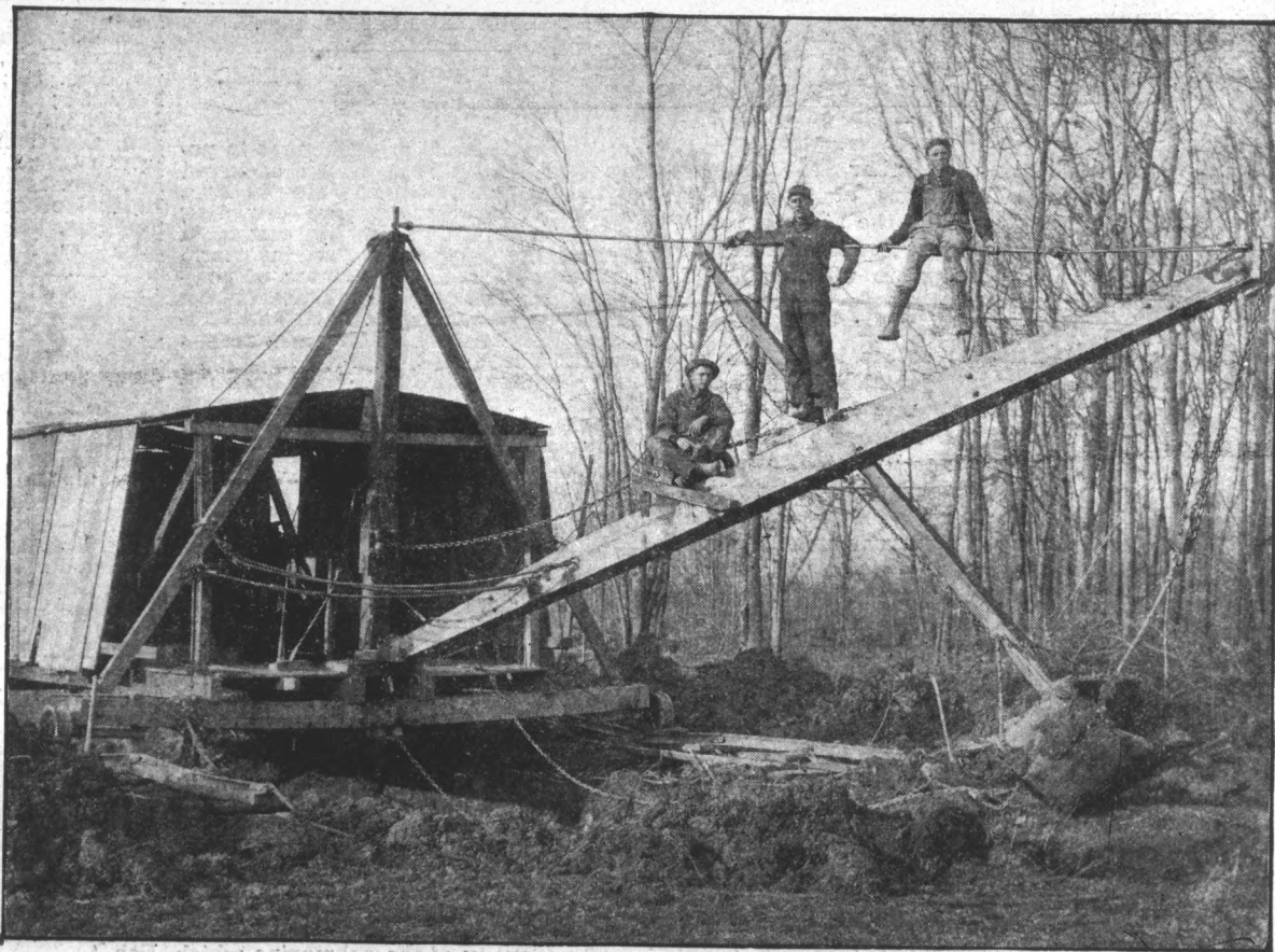
Dredging an Outlet for Tile Drainage in a Low and Level Section of Michigan.
