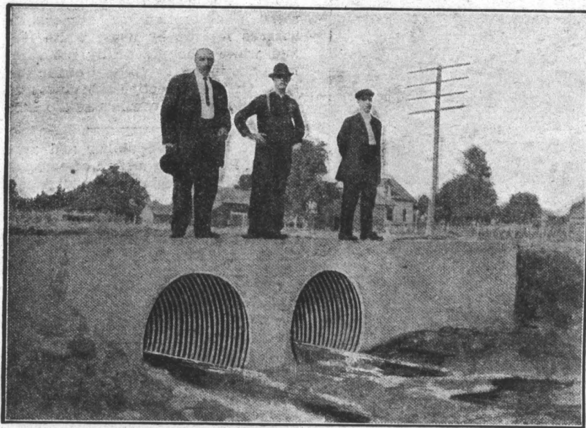
Corrugated Metal Culverts Set in Concrete Walls Insure Permanence at Low Cost.
