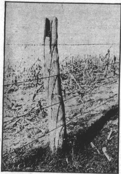
Fence Posts Made of Perishable Woods Should have the Tops as well as the Ground Portions Treated. (la. Ex. Sta. Photo).
