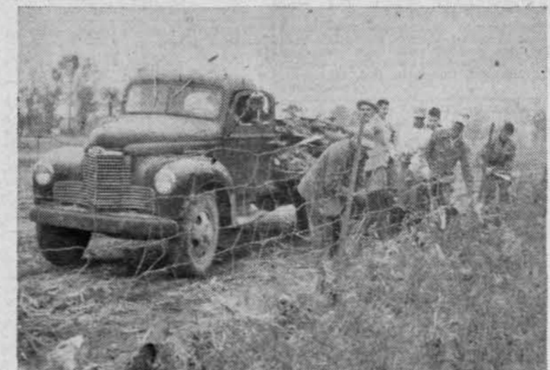
Fences Left Standing were Torn and Laden with Junk
