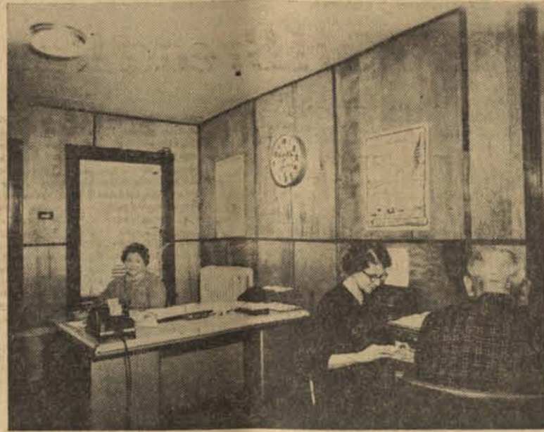
Barry County Farm Bureau Offices
