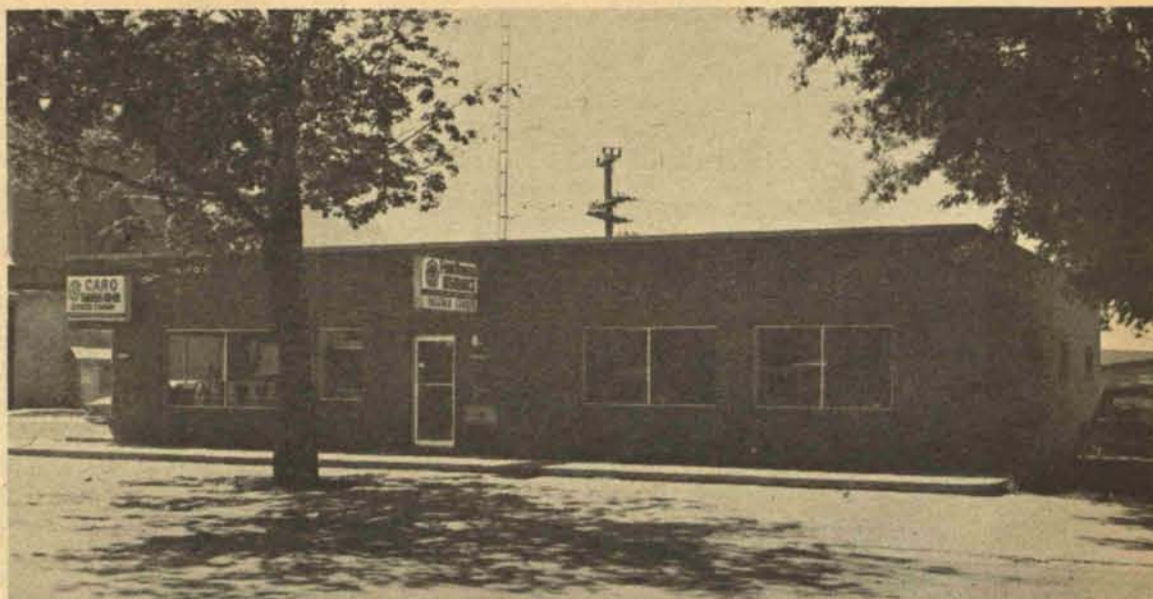
JUSTLY PROUD of their spacious new quarters, Tuscola County Farm Bureau members built this Farm Bureau Center. The office building neighbors with the Caro Farmers Cooperative Elevator and the Farmers Petroleum Cooperative branch for the county—both dispensing Farm Bureau supplies.
