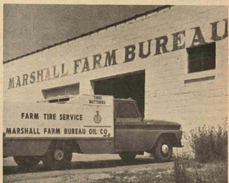
EVEN A MODERN TIRE service truck goes to the farm from the up-to-date Marshall cooperative location. A fully modern gasoline service station is well patronized by residents of the area. Even wheel balancing is included.
