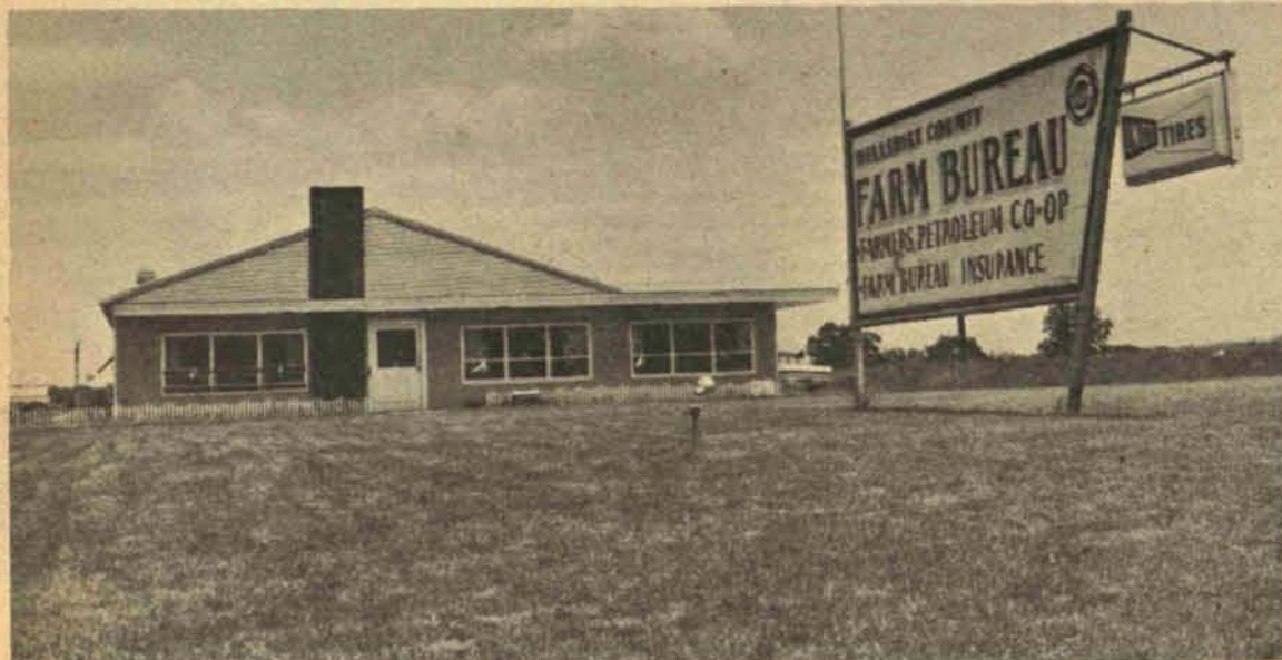
EYE APPEAL AND SERVICE. The Hillsdale County Farm Bureau sign tells the story that makes this a service center. Behind the office is a warehouse of the Farmers Petroleum Cooperative. Farm Bureau people of Hillsdale county built this office in 1960. The bank of windows at the right looks into the specially-planned meeting room. Service companies help finance the office operations.
