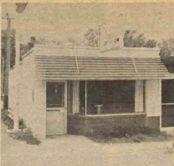
PURCHASED AND IMPROVED by the volunteer work of St. Clair County Farm Bureau members, this office serves the county with efficiency. Located at Memphis.
