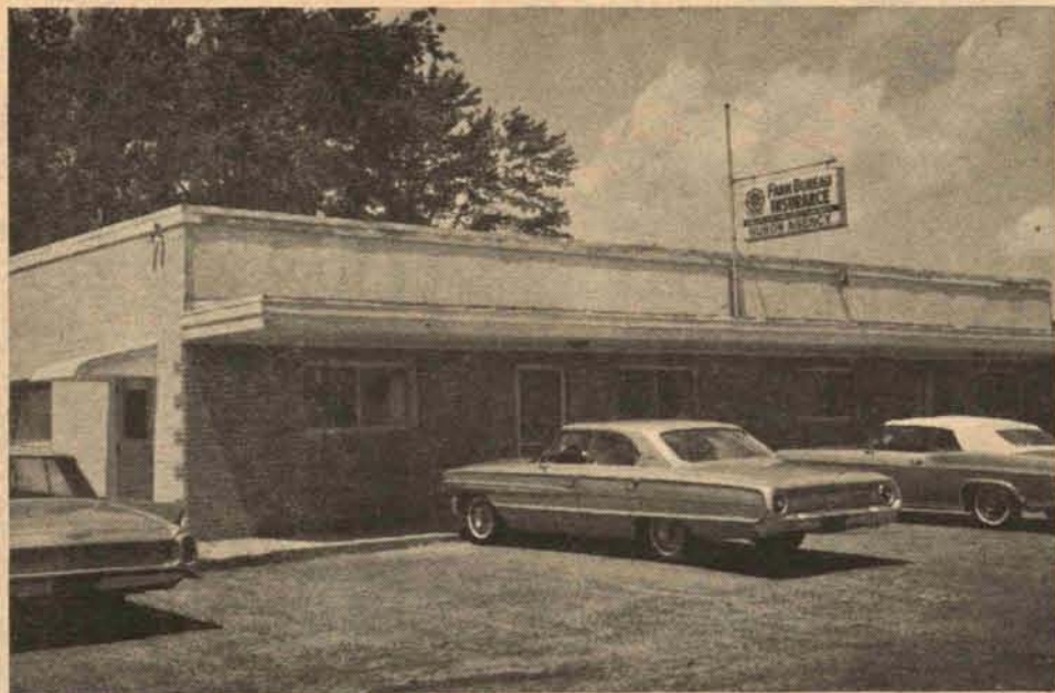
WHERE PEOPLE GATHER for business and trade. Huron County Farm Bureau owns part of a shopping center. Facilities include kitchens and a large meeting room. The office has "increased traffic 250%", says the county Secretary.
