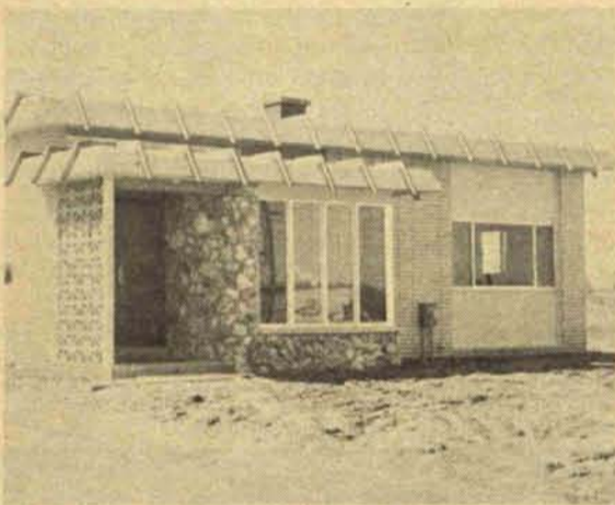
NEW OFFICE QUARTERS—for the Isabella Farm Bureau, at 1019 N. Mission Street, Mt. Pleasant. For the past 12 years the office has been located within Farm Bureau Services elevator and retail store buildings on the city's west edge. The new office is shared with the Production Credit Association, and contains a board-meeting room and kitchen.
