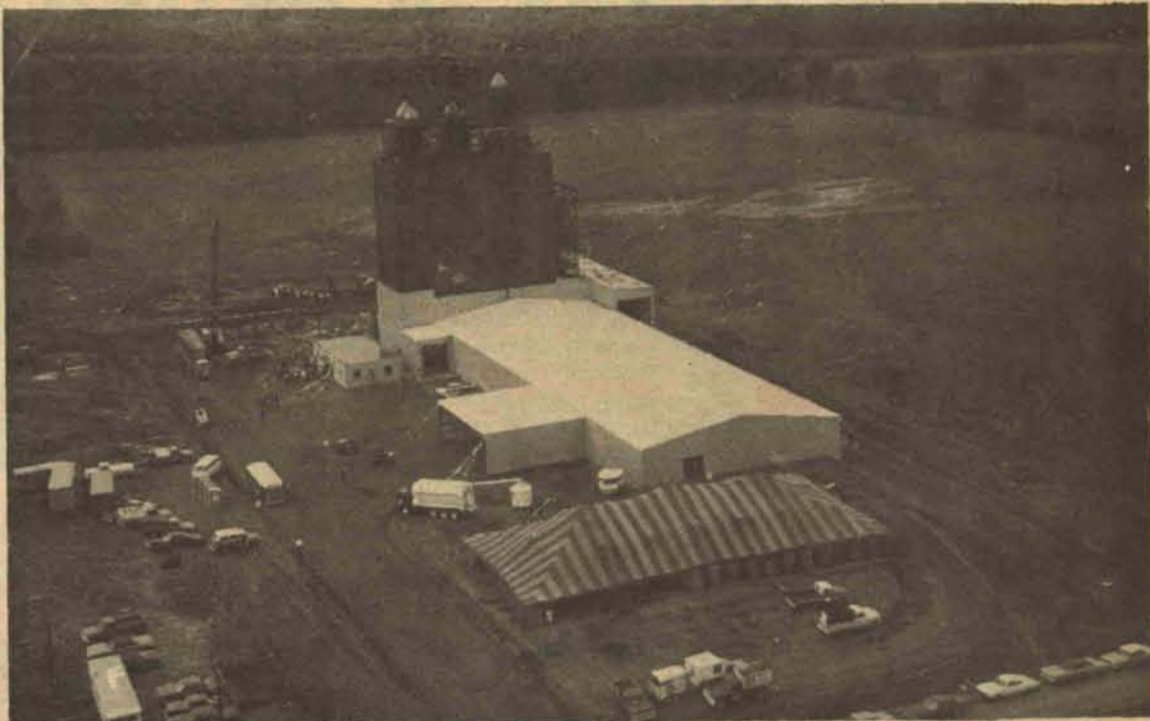
HELICOPTER'S-EYE VIEW — of Farm Bureau Services new million-dollar-plus feed plant provides an idea of the size of the involved area and the potential industrial park growth-area around it. Off-site parking handled the many hundred cars, with participants bussed to the plant site.
