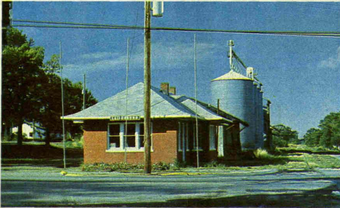
Laingsburg's permanently closed rail station and paved-over tracks stand as reminders to the impact of rail line abandonment. The grain storage facilities in the background are a part of Ovid Roller Mills, which formerly shipped grain on the now defunct Penn Central's line from Lansing to Owosso. The State of Michigan subsidized this line for awhile, but soon found that allotted funds had to be diverted to keep other, more heavily traveled sections of track open. After the State withdrew its support, the mill was forced to ship grain by truck at additional expense.
