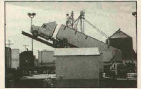
Pioneer customers and other curious farmers had a chance to see the inner workings of one of the Midwest's largest seed processing facilities, from unloading semi trucks filled with seed stock still on the ear through the massive dryers and bulk storage.
