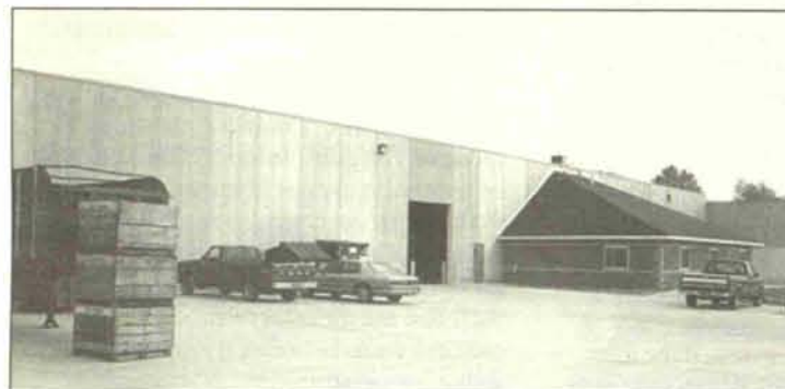
The 400-foot-long cement building located in Sparta provides an affordable structure for the growers to build their $2.1 million facility. It also provides the ability to expand by adding on to the existing facility.
