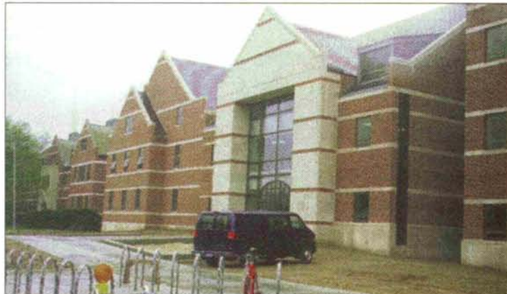
Anthony Hall underwent extensive renovations as part of the initiative.
