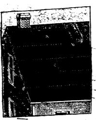
The method of "unrolling" and laving the felt. B-Showing "lap" of top width over lower one. C-Showing "splice" of the D=Fastening of the felt with worden cleats" at eaves
