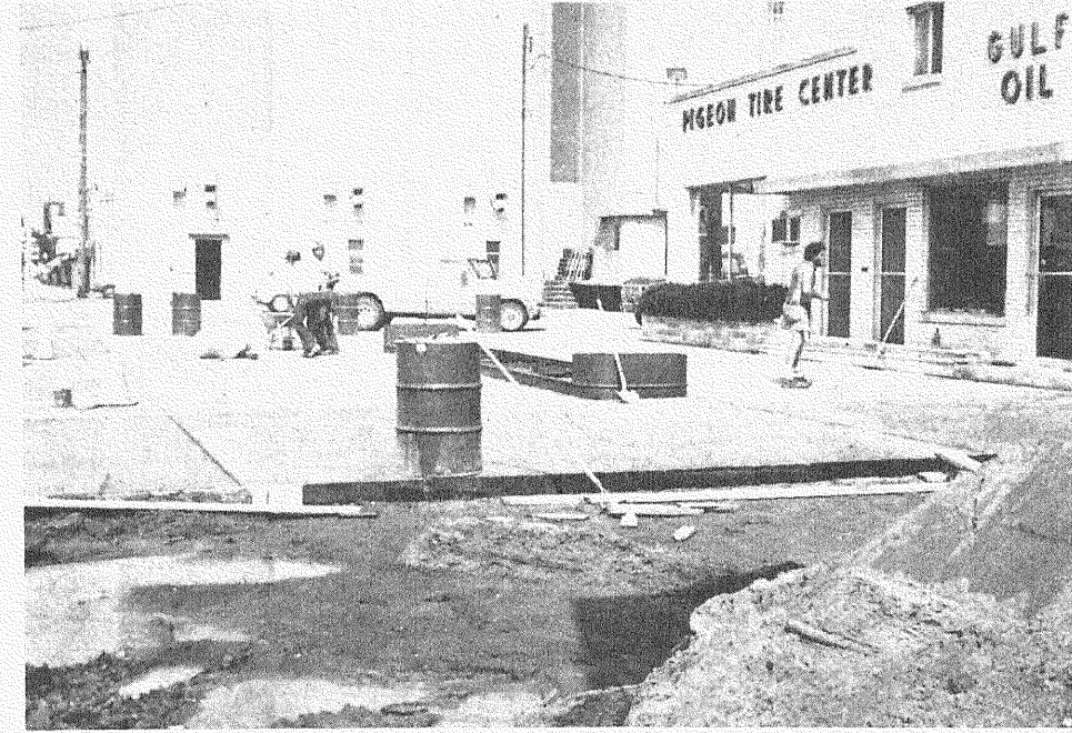
NOW THE CONCRETE WORK is nearing completion, with gas tanks installed underground. Pumps are expected to be placed in the concrete next week, with customers invited to patronize the revamped station in the near future.
