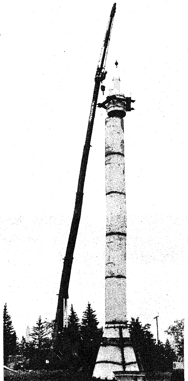
A NASA ROCKET? No, Pigeon's new water tower is taking shape west of town, as workers prepare to add the round tank on top. RICH SWARTZENDRUBER PHOTO
