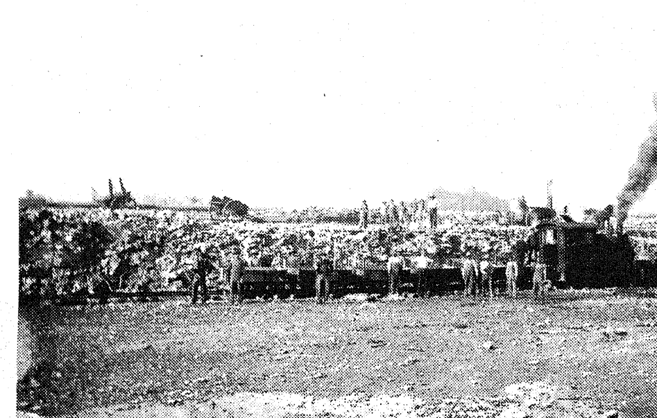
ANOTHER METHOD OF LOADING: a locomotive pulled the cars instead of horses and mules. Dast remembers when dirt on the stone was all removed by hand.
