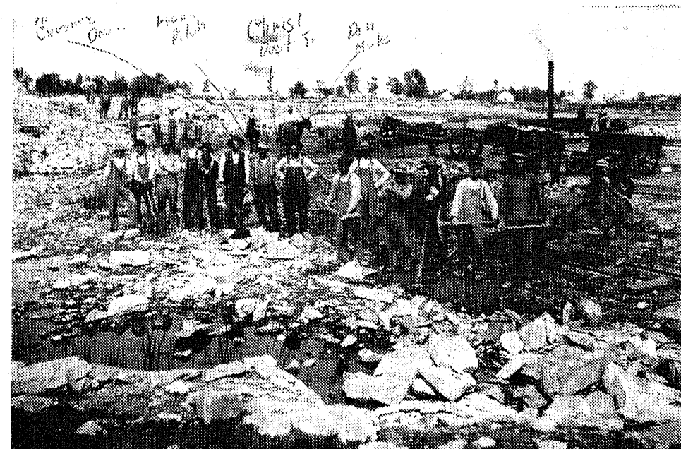
QUARRY WORKERS loaded carts on the right side of the picture, then moved them to railcars which were pulled by horses and mules. This photo is from 1910 or earlier.
