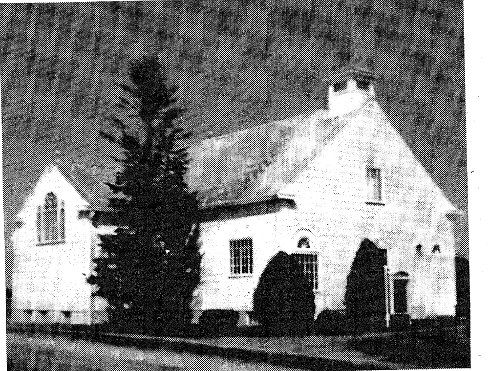
CHANDLER PRESBYTERIAN CHURCH, as it stands today . . .
