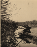
SCENE ON THE BRIDGE NEAR FREDERICK.
