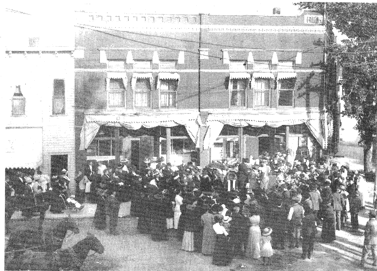
HERE'S HOW Downtown Sebewaing's Myers & Riedel store looked 100 years ago, in this photo from Alice Fauser's collection. The picture was likely taken during the store's grand opening in 1895.
