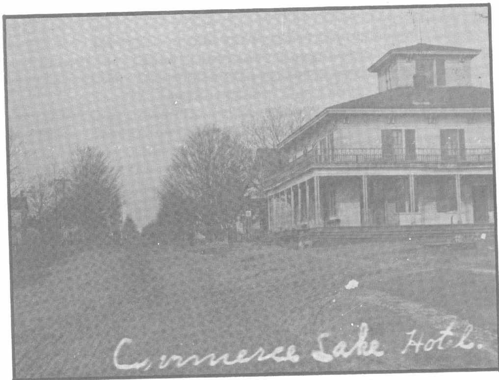
Looking west on Commerce Road.
