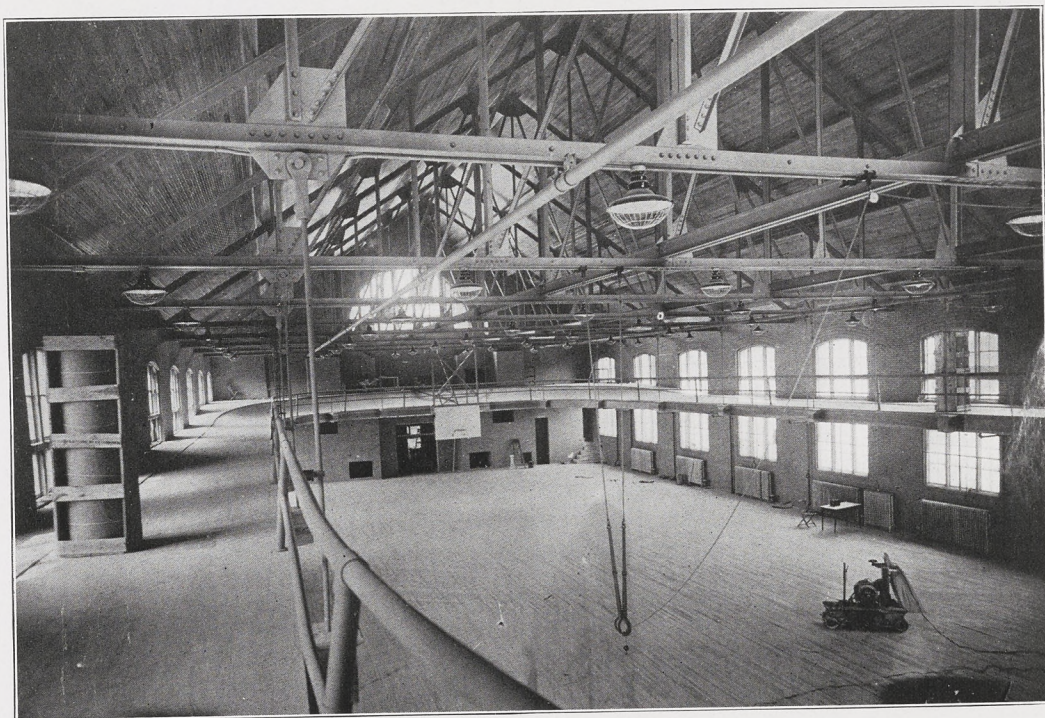
THE LARGEST GYM FLOOR IN THE STATE (Before Completion)
