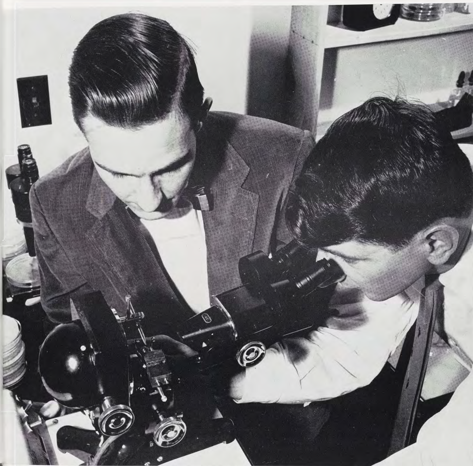
Mycology students Fred Van Nostran and Ed Tylutki make a very minute point on a glass needle on the Microforge. This needle, one-ten thousandth of an inch in diameter, will be used for picking up single spores in experiments on fungi which they are conducting.
