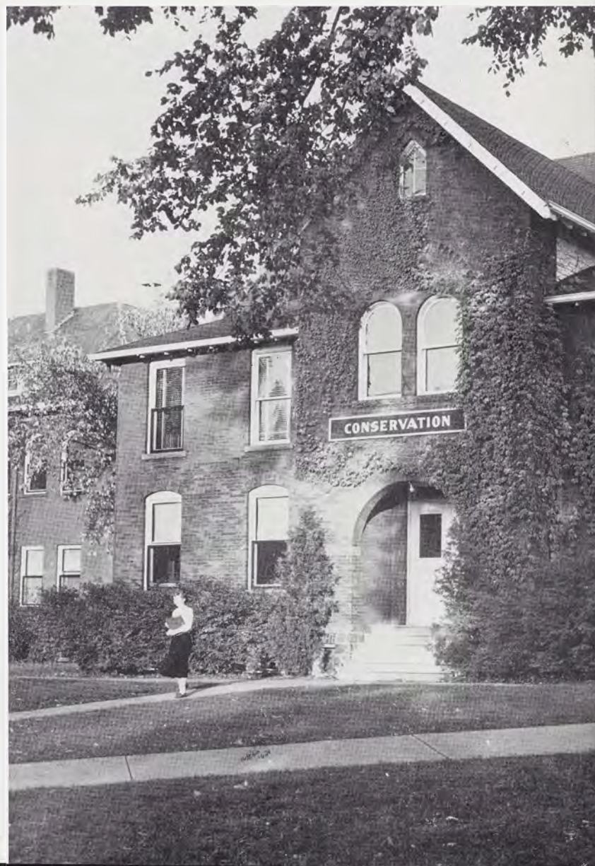
Red-bricked, ivy-walled Conservation building, 1955.
