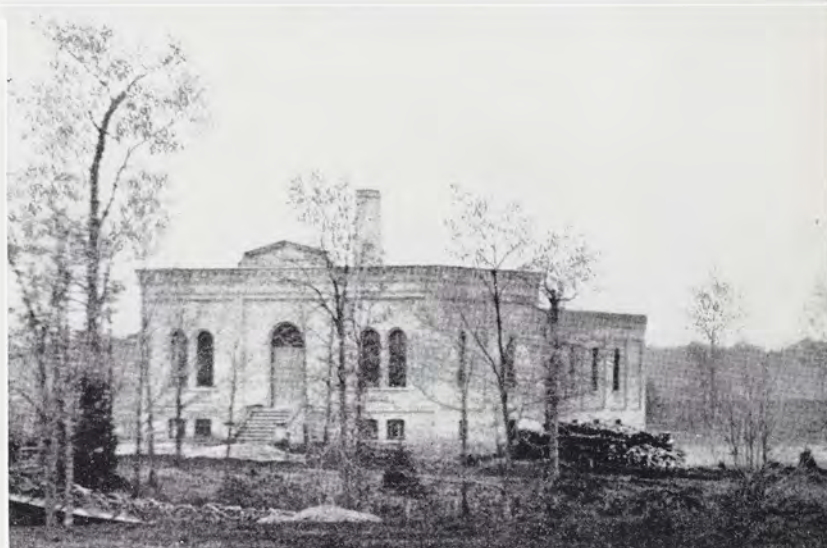
The "Chem Fort," two years old in 1873. A pile of firewood anticipated winter. Footbridge, left, spans gully.
