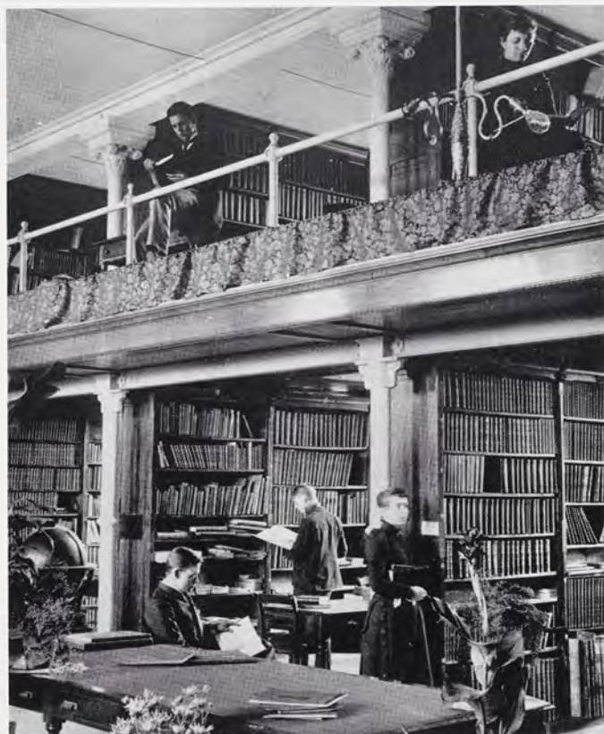
The library was the second building on campus to have electric lights (1890). The yellow light of carbon filaments left much to be desired, however.
