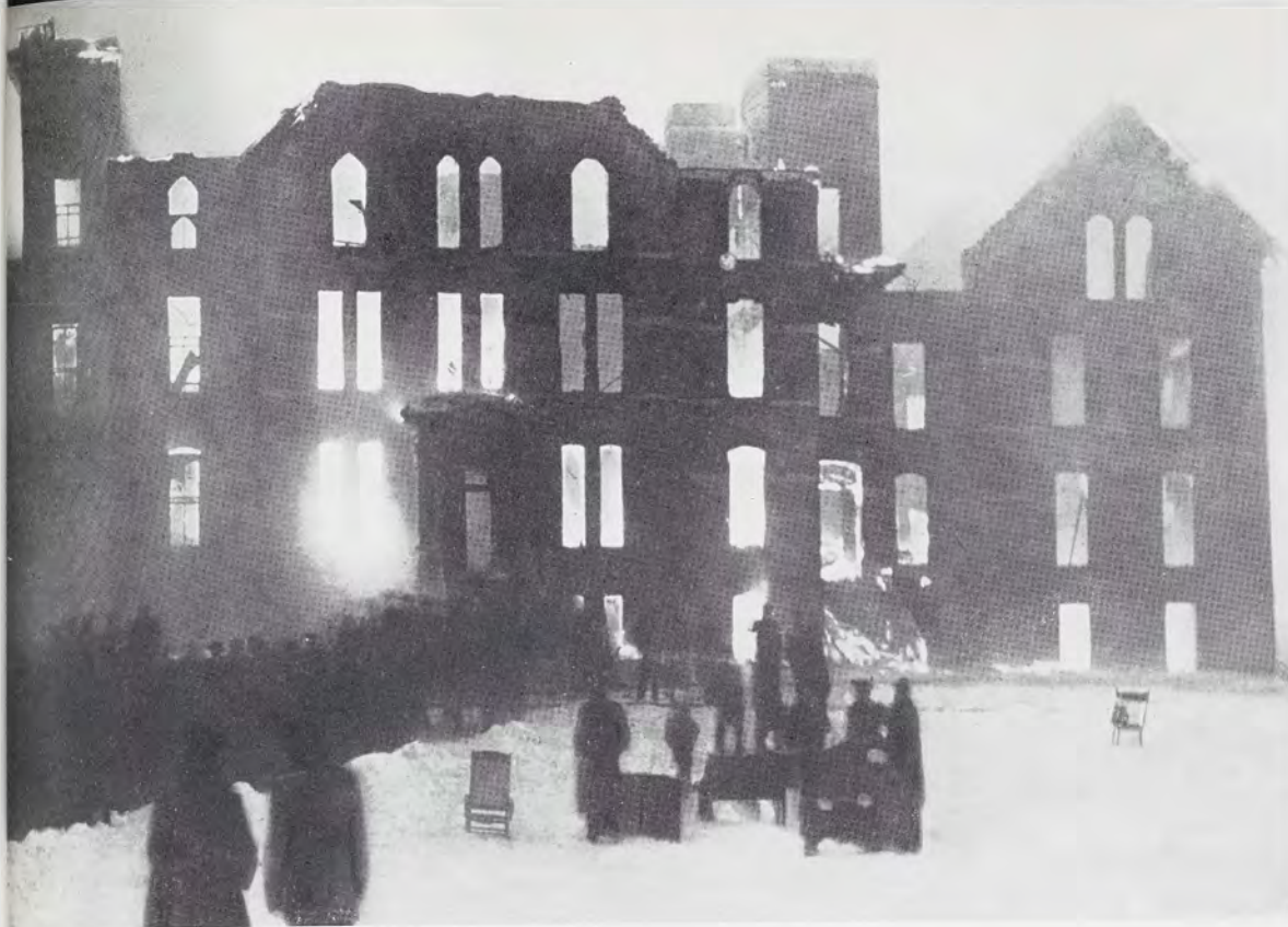
By 6:30 a.m., Feb. 11, 1905, only a few glowing bricks were left of the first Wells hall. A new Wells—the present one—was built quickly to replace it.
