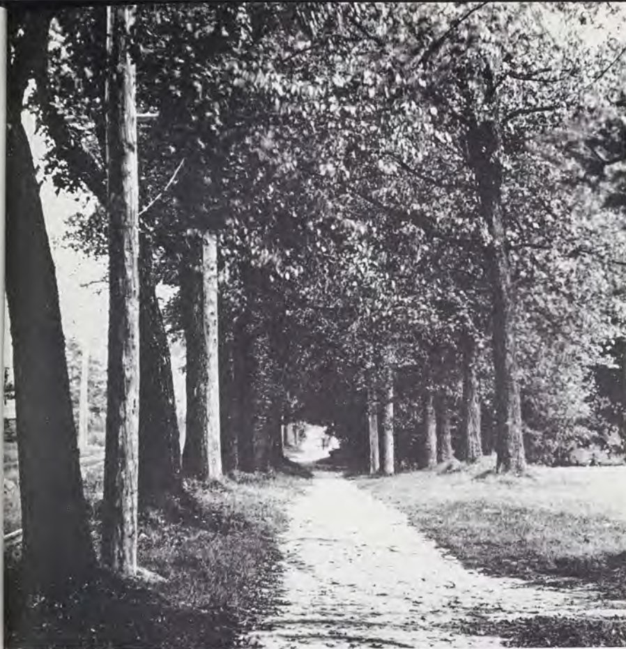
The shaded bypath on Michigan avenue invited strollers, whizzing cyclists. Trolley tracks, left, were laid in 1894. Looking east, about 1900.
