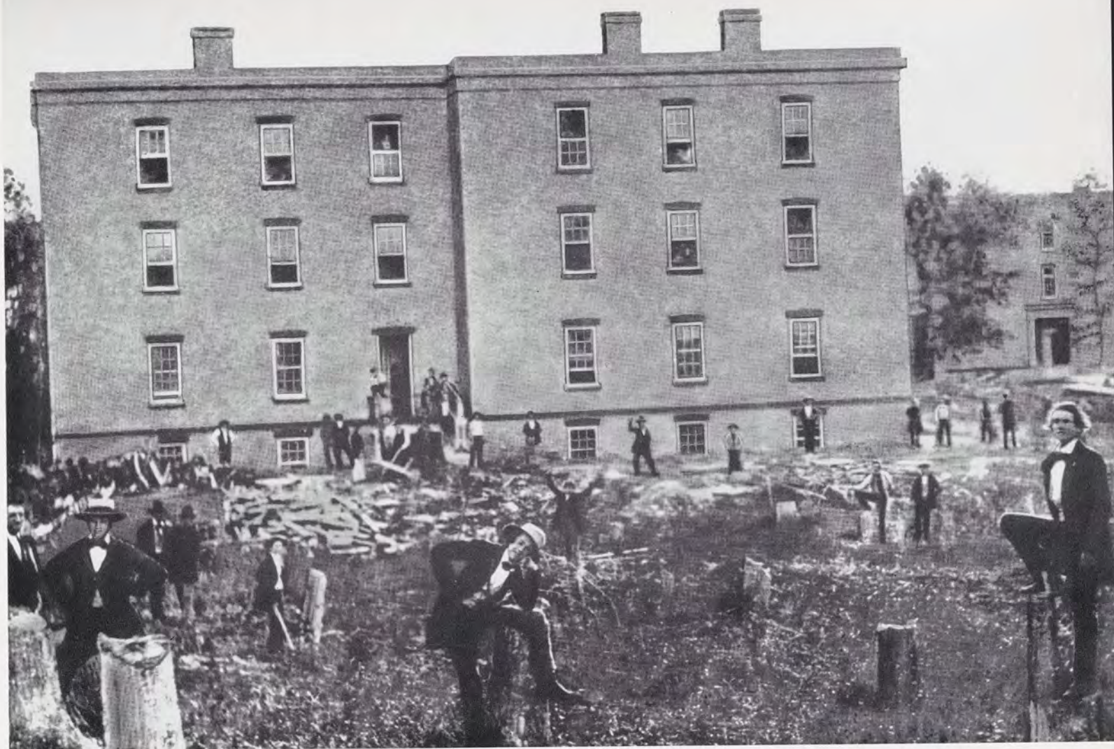
Workers rushed to complete the boarding hall, Saint's Rest, for the college opening in the spring of 1857. Stumps were left for the students.
