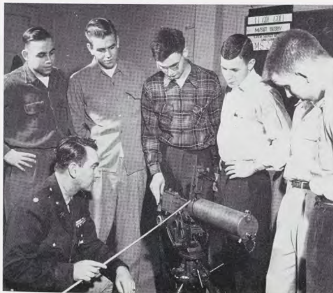
An Army instructor points out the important features of a .30 cal heavy machine gun to sophomore cadets. A course in crew-served weapons is part of all students' training.
