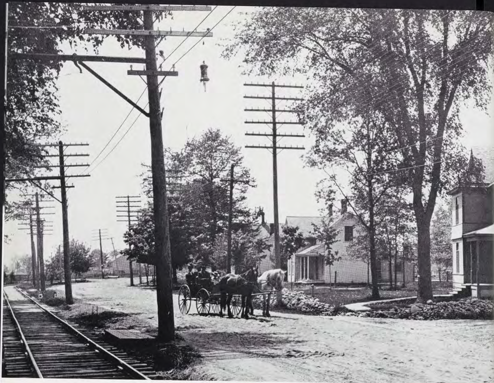
Newly-laid trolley car tracks, 1896, lead from the Beal street entrance on campus toward Lansing. A ride cost a nickel. The trip to town took 15 minutes, but passengers were expected to help put the tram back on its tracks when it jumped off.
