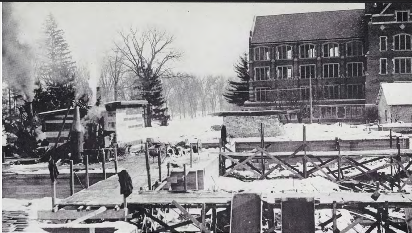
Construction of the $300,000 Memorial Union building in 1923 was a combined student-alumni-faculty effort. It was dedicated to World War I soldiers. The new Home Ec building, background, is not quite complete.
