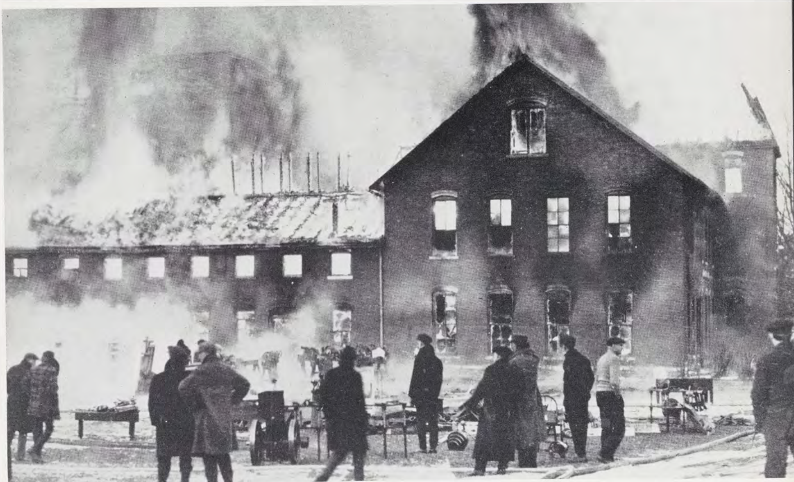
Firemen and student volunteers were able to save little equipment when the historic Mechanical Laboratories were destroyed, along with Engineering building, on the eve of America's entry into the World War.
