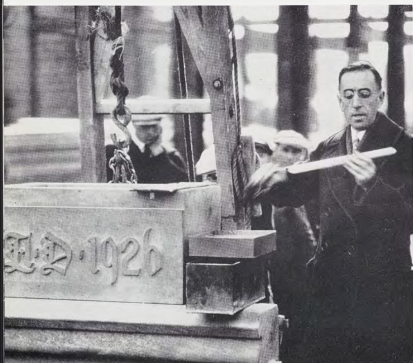
A. J. Clark, head of the chemistry department in 1926, laid the cornerstone of the Kedzie Chemistry building.
