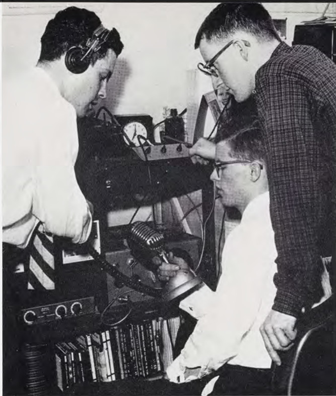
Jim Taggert, Bill Lewis and Jack Grenard examine the tape recording intercom system which they have installed to communicate with other rooms in the dormitory.
