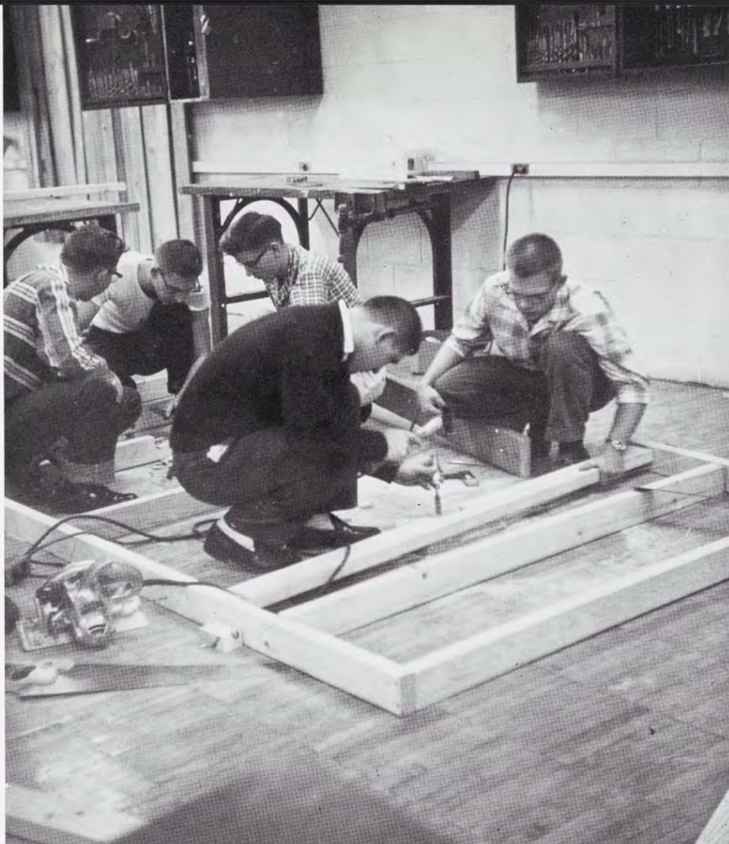
Agricultural Engineering students construct a wall section for a portable farm building.
