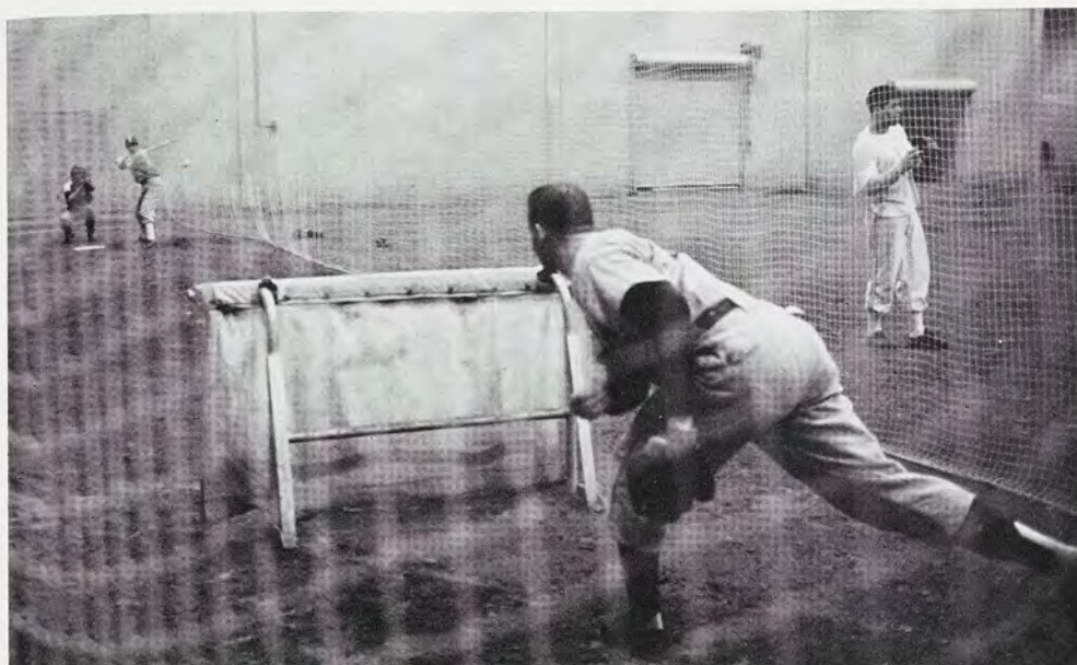
The dirt arena enabled the baseball team to hold indoor winter workouts.
