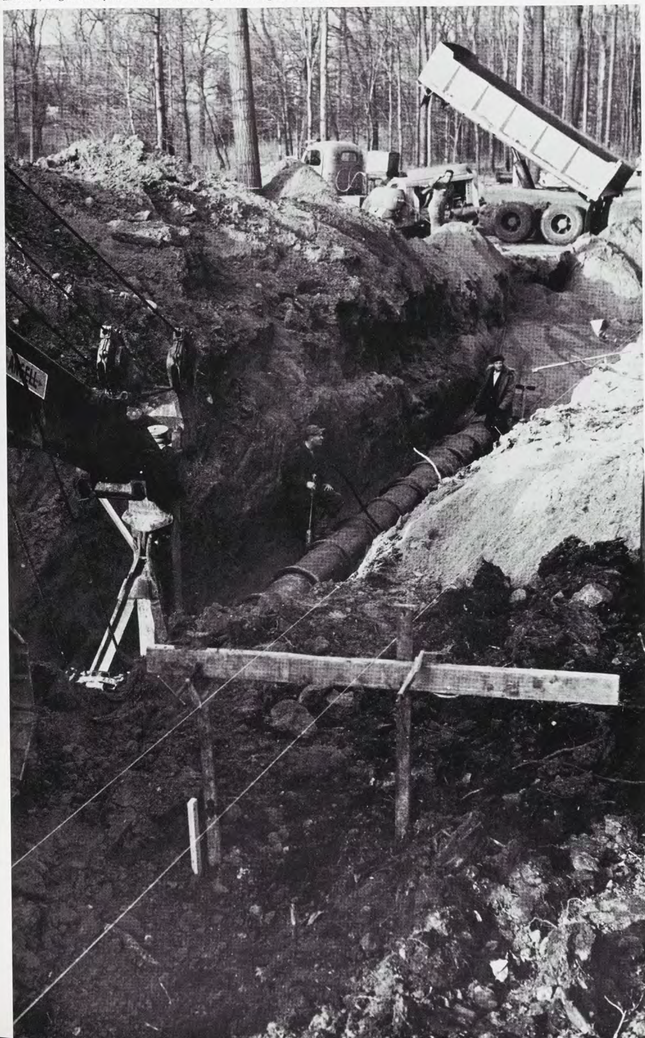
Construction on a new graduate dormitory, located near Van Hoosen, began this year. The dorm is expected to open next fall.
