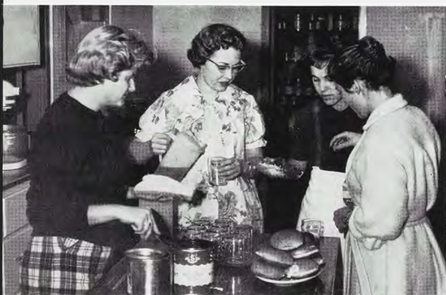
The cook's night out means kitchen duty for the ZTA actives.
