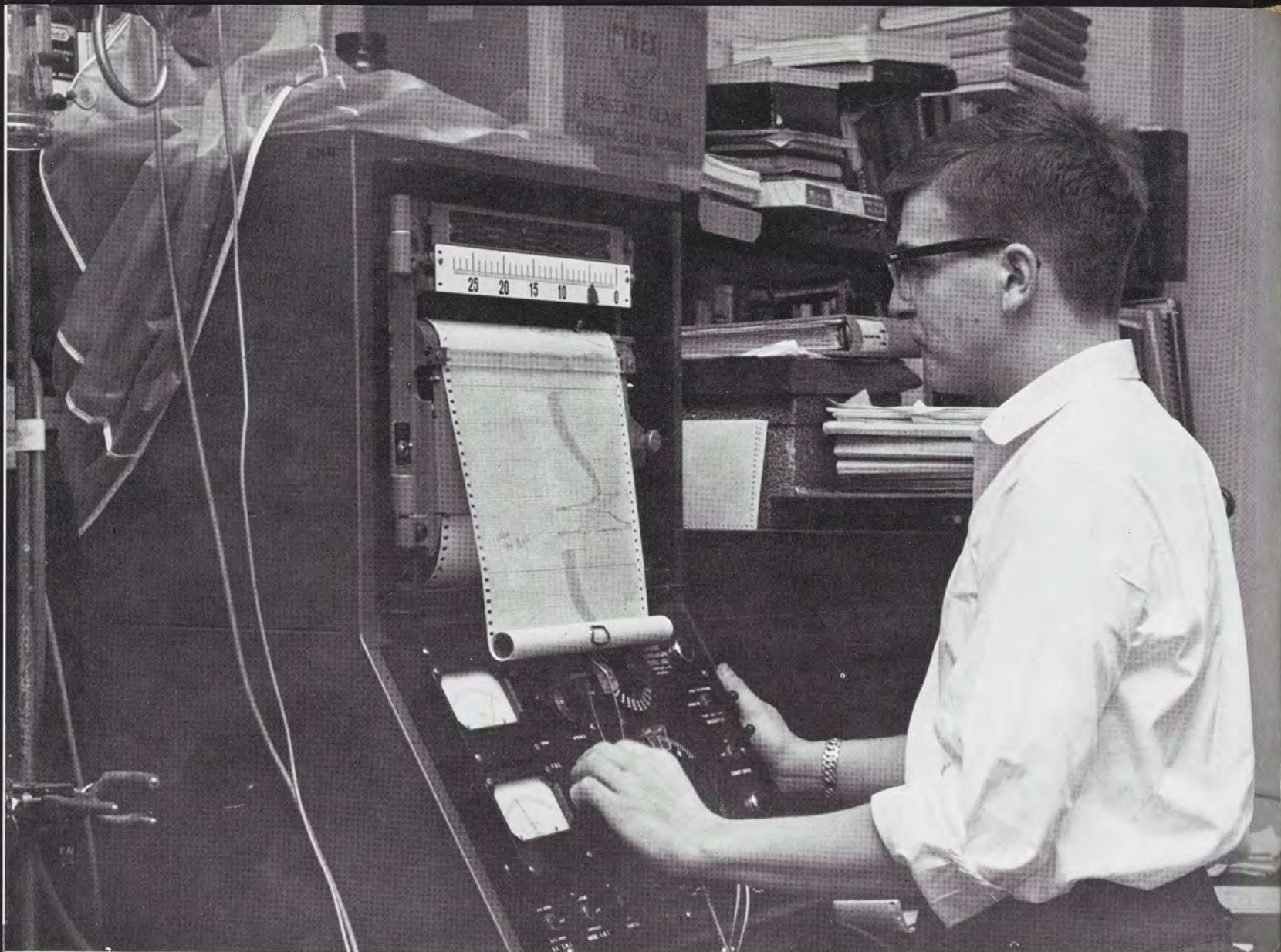
Norman Fishel, Honors College sophomore, operates a polarograph for his original research project in the analysis of chloramine.
