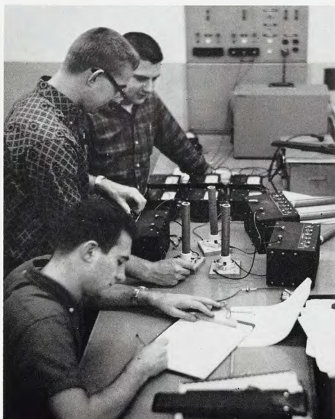
A group of electrical engineers measure the resistance of an electrical circuit.
