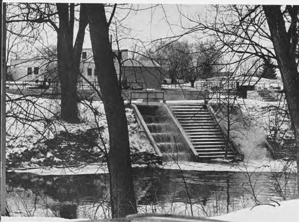
The sewage plant, a source of constant complaint, is being moved this summer.
