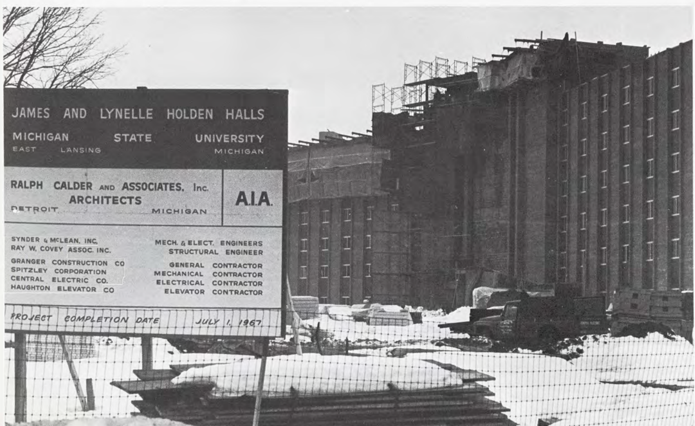
As the year progressed, work on Holden neared completion.
