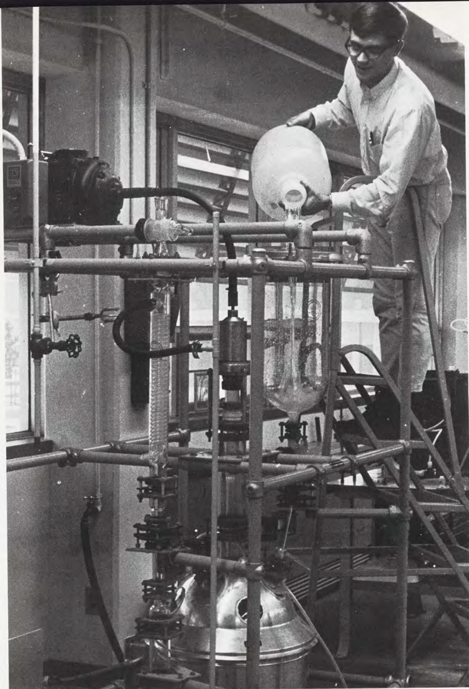
An experiment in fluid dynamics teaches the relationships of pressure and fluid flow.
