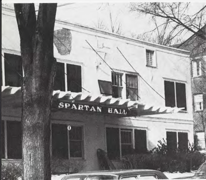
A typical supervised residence.
