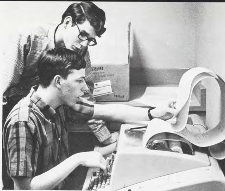
The students in Briggs quickly become familiar with all the elements of computer operations. They have available to them several key punch machines as well as a direct link with the computer which permits instantaneous response to student-written programs.
