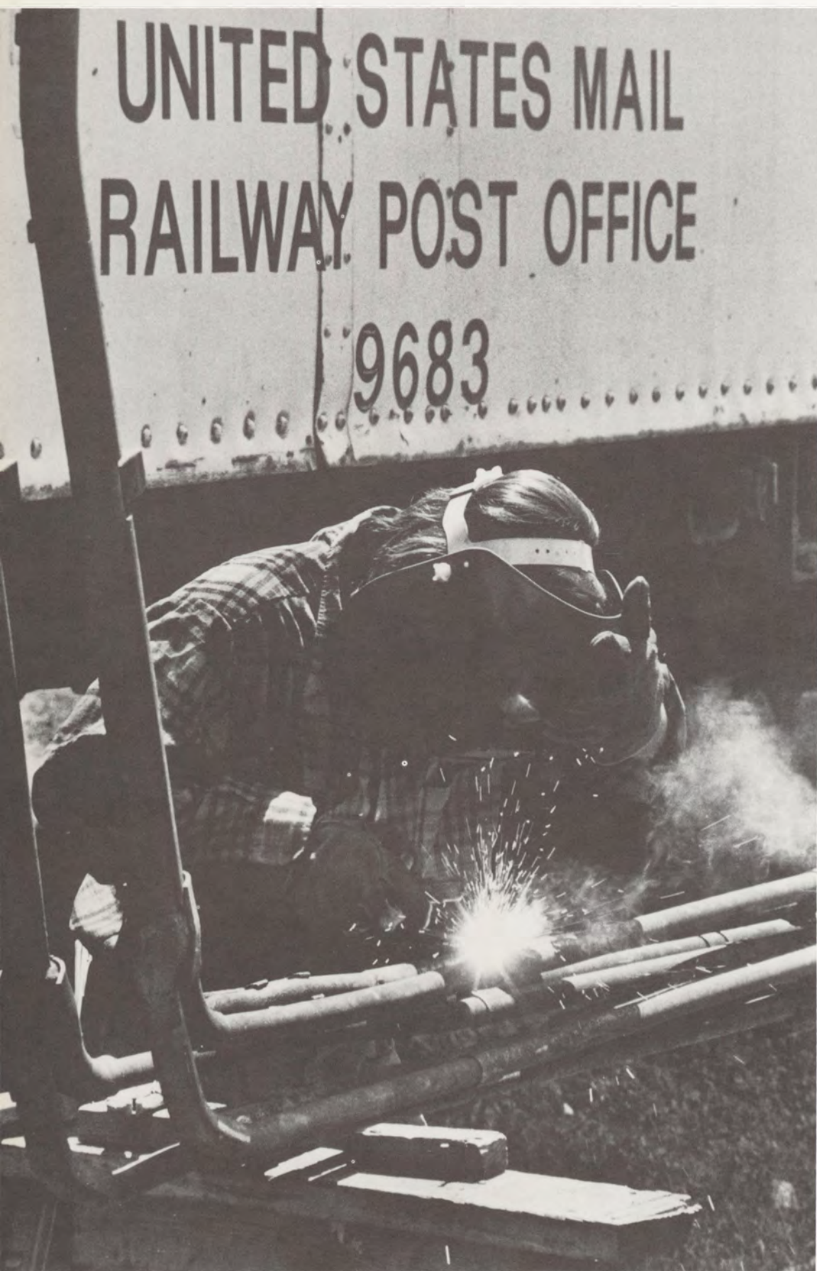
New superheater pipe is welded into place by Charles Julian, a graduate student in Geology.
