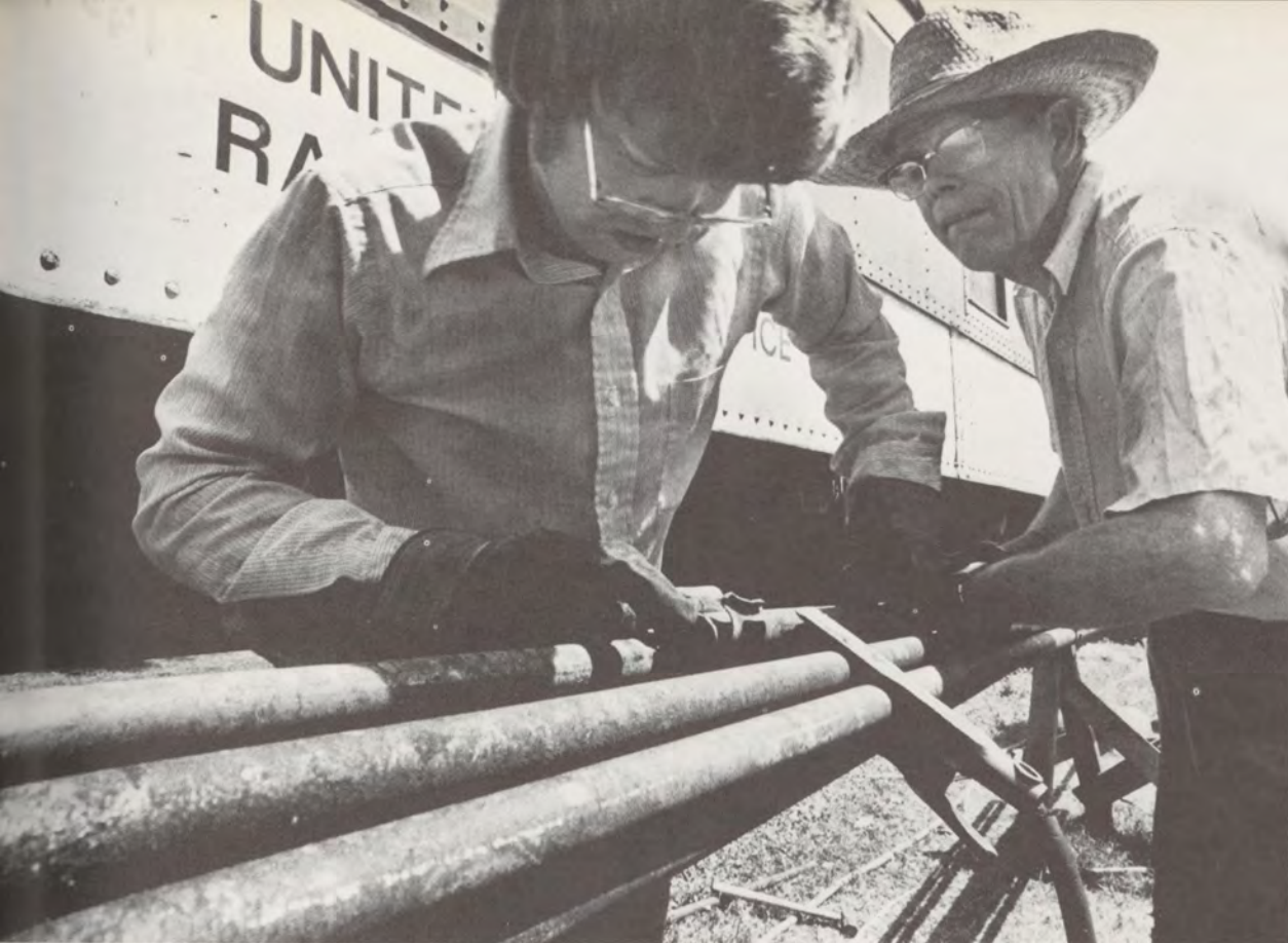
Wendell Sturges of the MSU Grounds Maintenance Department helps Dean Eicher (left), coordinator of undergraduate physics labs, replace superheater pipe.
