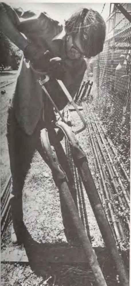
Defective superheater pipe is cut out by MSU graduate Roger Scovill (above). Roger Scovill and David Jones check superheaters for leaks.
