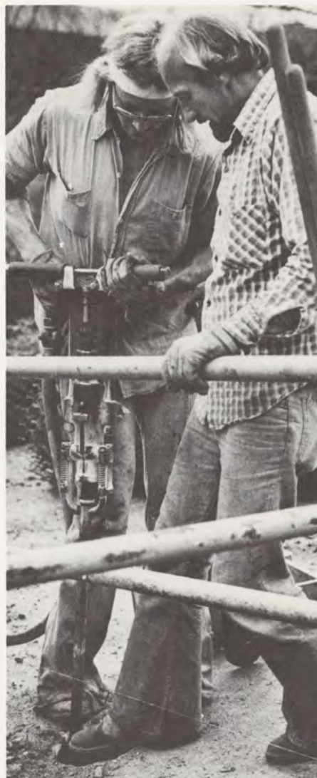
Workers drill holes for new rails.
