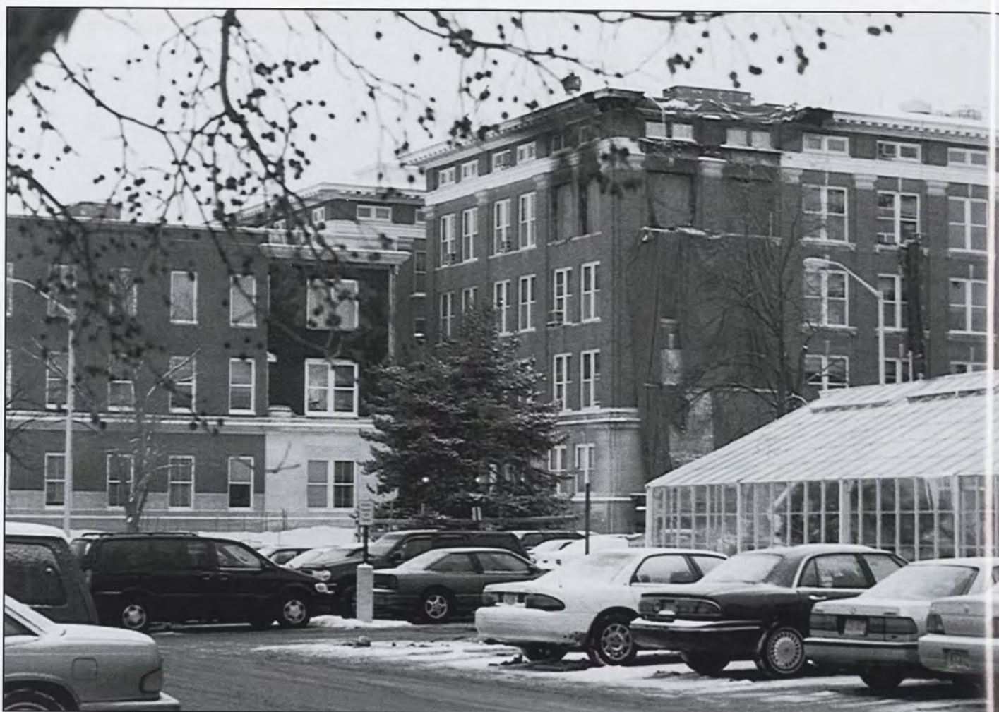
December 31, 1999, the Agriculture Hall was set on fire due to protest of cloning vegetables. Workers put in endless hours trying to put the oldest building back to its normal state.
