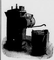
Are you interested in Acetylene Lighting? If so, write us. The Cline Machine has stood the test of two years' service. It is perfectly automatic. There are no valves in its construction. Has compartment Generator. There is absolutely no loss of gas through the blow-off. If you want the best, up-to-date machine, write the
