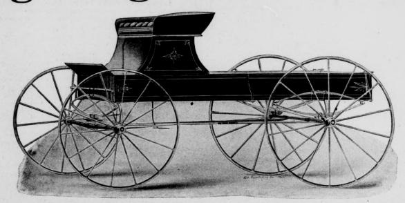
The above represents our No. 52 Delivery Wagon, which is especially adapted to meet the requirements of the grocery trade. Capacity 1,500 pounds. Write to us for catalogue and prices.
