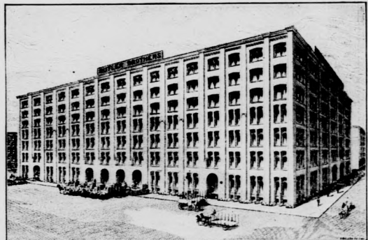
Shipping Warehouse, St. Louis
