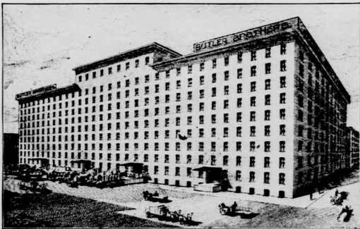
Shipping Warehouse, New York
