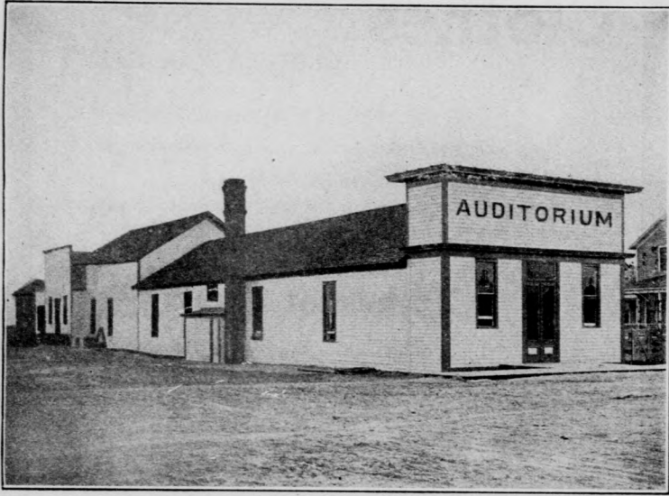
THE OLD STORE, NOW USED AS OPERA HOUSE.
