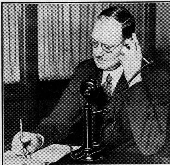
Graham-Paige officials use the telephone to call former employees back to work
