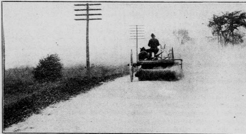
Oiling N. Canal St. May 10, 1910 City sweeper preparing road surface for application of oil
