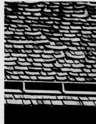
Wood Shingles After Five Years Wear
