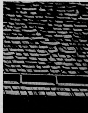
Wood Shingles After Five Years Wear
