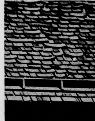
Wood Shingles After Five Years Wear
