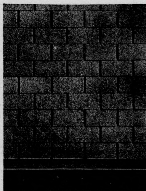
Reynolds Slate Shingles After Five Years Wear
