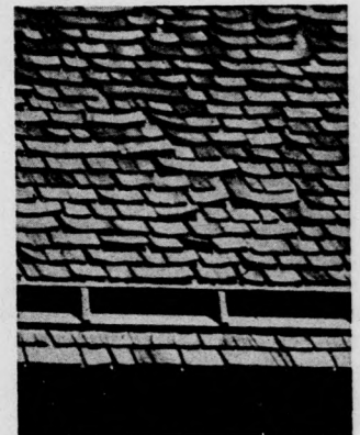
Wood Shingles After Five Years Wear
