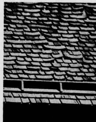
Wood Shingles After Five Years Wear
