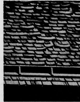
Wood Shingles After Five Years Wear
