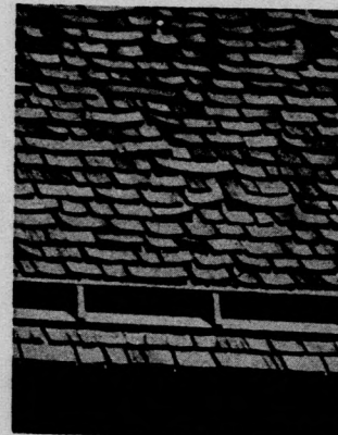
Wood Shingles After Five Years Wear
