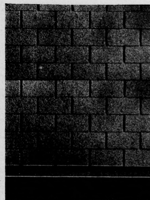
Reynolds Slate Shingles After Five Years Wear
