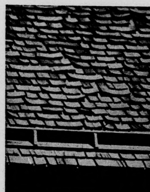
Wood Shingles After Five Years Wear
