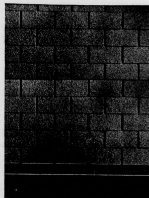
Reynolds Slate Shingles After Five Years Wear
