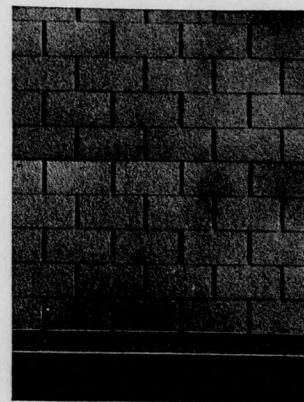
Reynolds Slate Shingles After Five Years Wear
