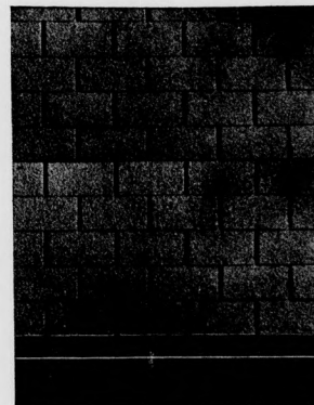
Reynolds Slate Shingles After Five Years Wear
